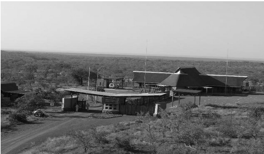
Establishment of Border Post Between Kruger National Park (KNP) and Limpopo National Park (LNP)
